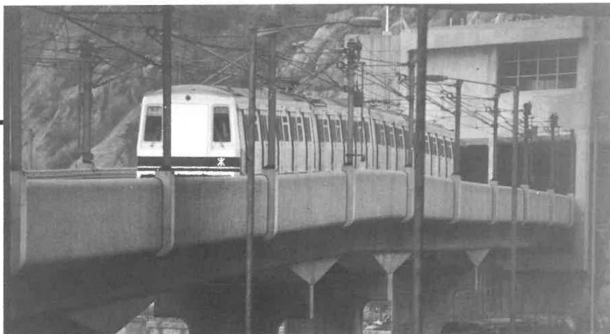
The extension of the Mass Transit Railway to Tsuen Wan costing $4,100 million, indicates good prospects for capital projects during 1980 and beyond.
